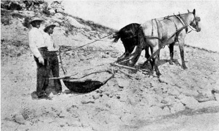
Figure 8. CMNH crew using a horse and scraper to remove overburden. Agate Springs Fossil Quarry, Nebraska. From Peterson (1906).
